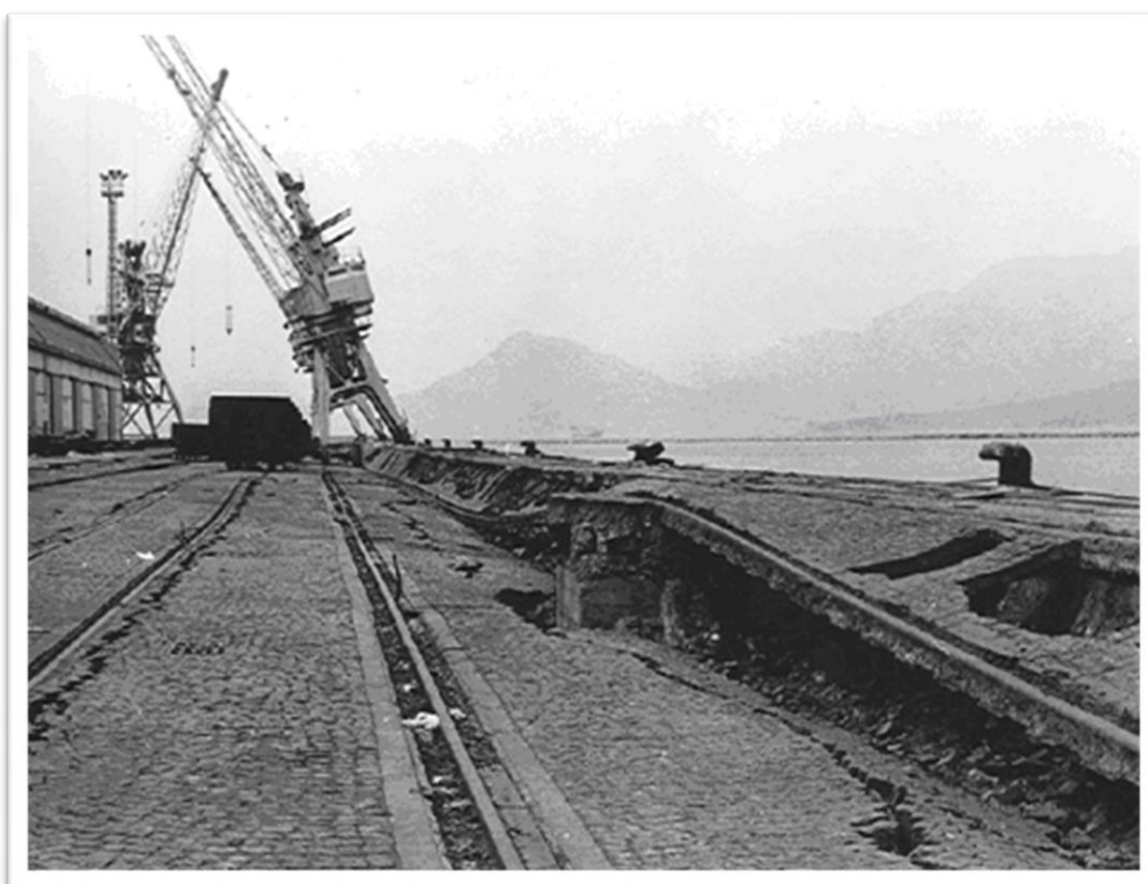
Crnogorski zemljotres 1979. - srušeni hotel Agava, velike štete u Luci Bar. Montenegro 1979 earthquake - Hotel Agava failure, extensive damages in Port Bar.
